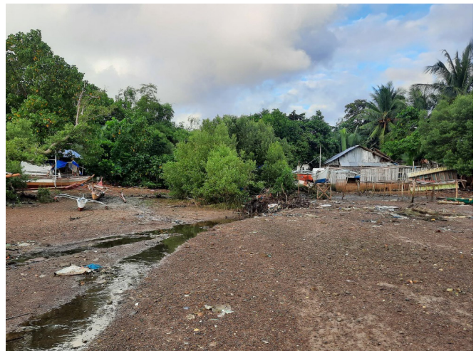
Treatment wetlands as secondary natural filter to STP discharge
