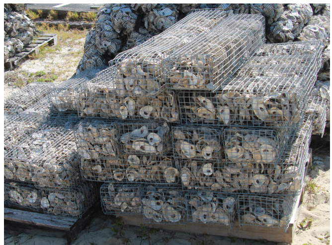
Gabion oyster baskets as breakwater to protect mangrove seedlings
