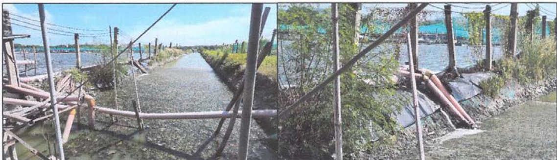
Outlet of the fishpens to settling pond and outlet to drain for BMW, O&B and Dos Aquafarm
