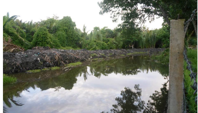
Accumulation of sediment and waste on waterways
