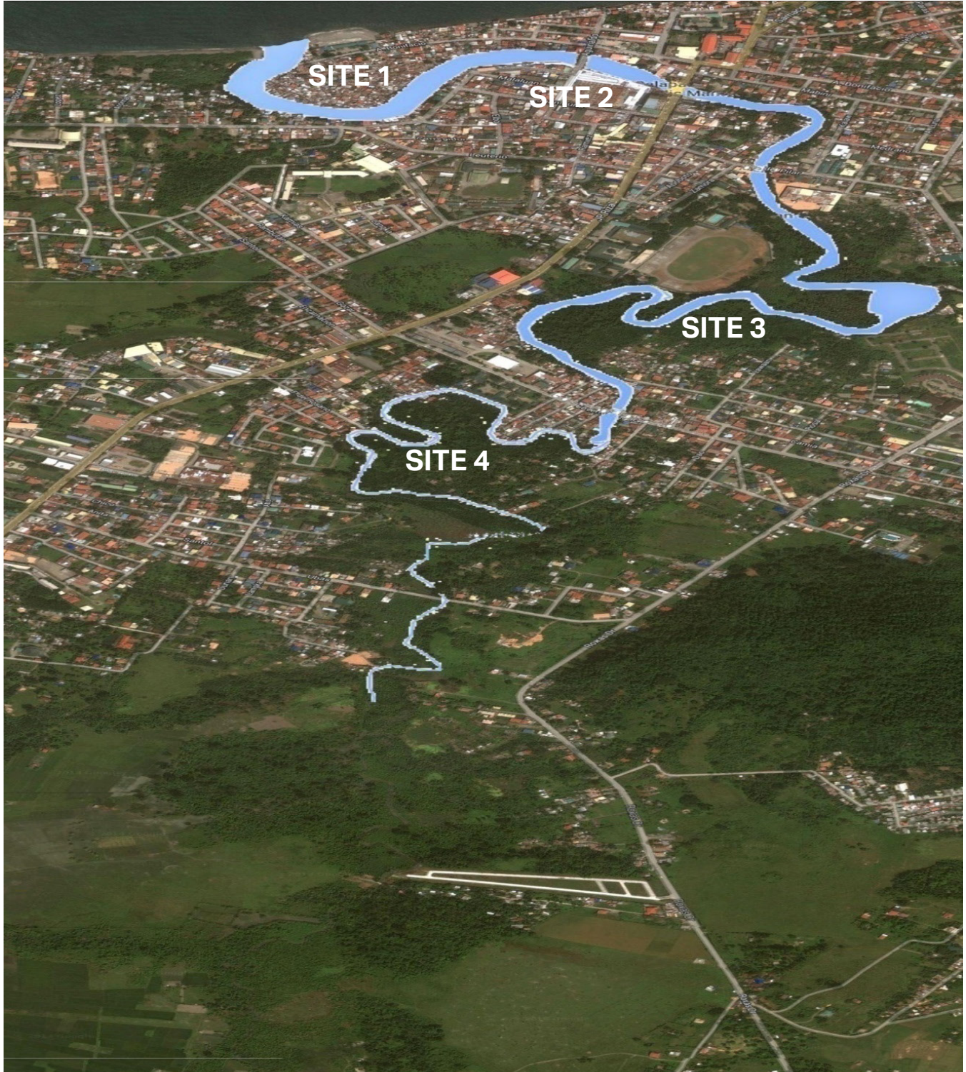
Sites 1-4 of Calapan City's Proposed River Rehabilitation and Eco-tourism Development Projects; Sites 3 and 4 proposed for inclusion in Green-Gray Partnership Project
