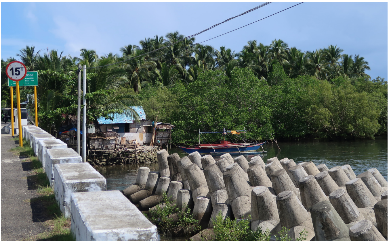
Existing tetrapods for protection of Borongan National Highway
