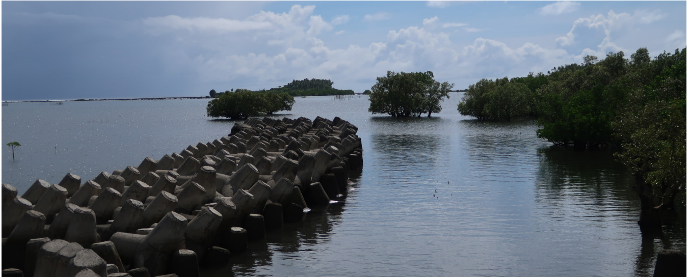
Existing tetrapods perpendicular to the Borongan National Highway for protection of mangroves
